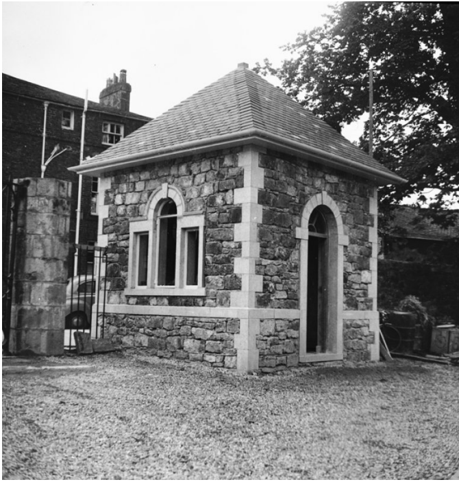
Fig. 6: The Beaumaris Castle Ticket Office photographed in 1954, from the D.O.E. Photographic Collection on Coflein (DI2010_2822.jpg).
